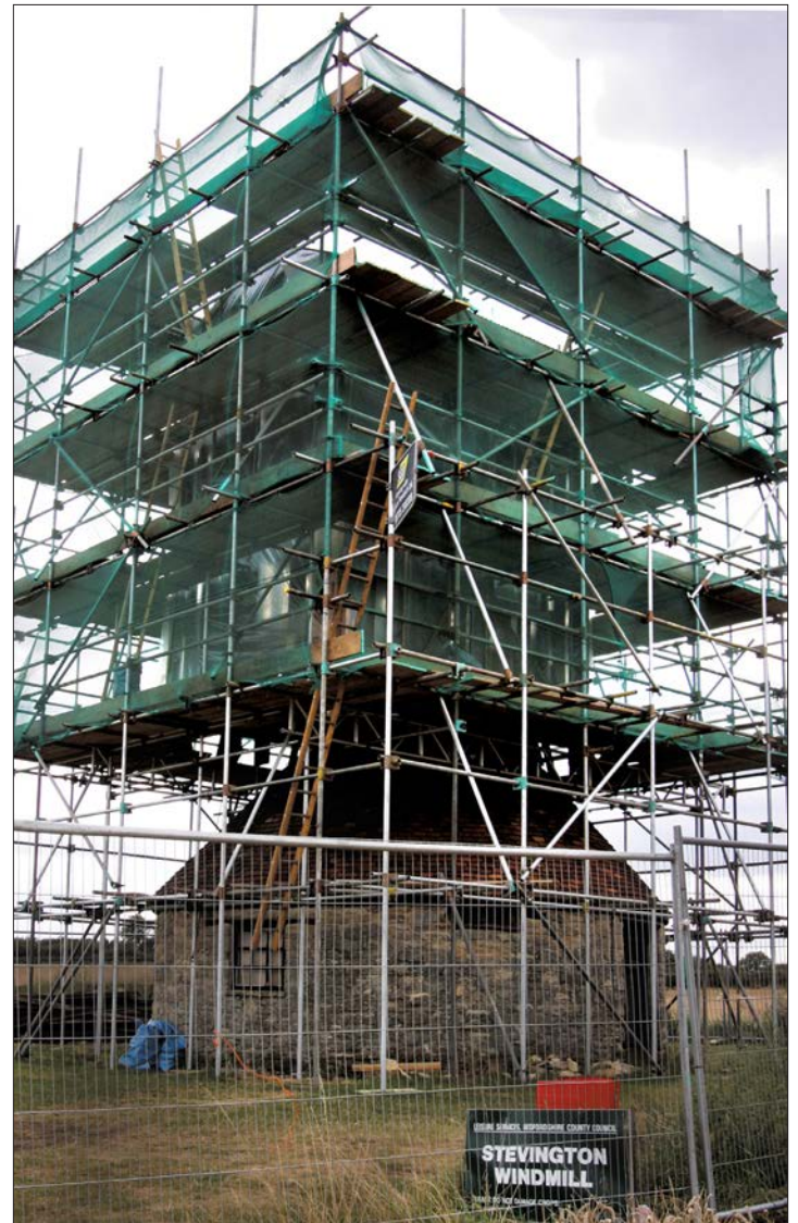
156 Mill work in Scaffolding 2003
