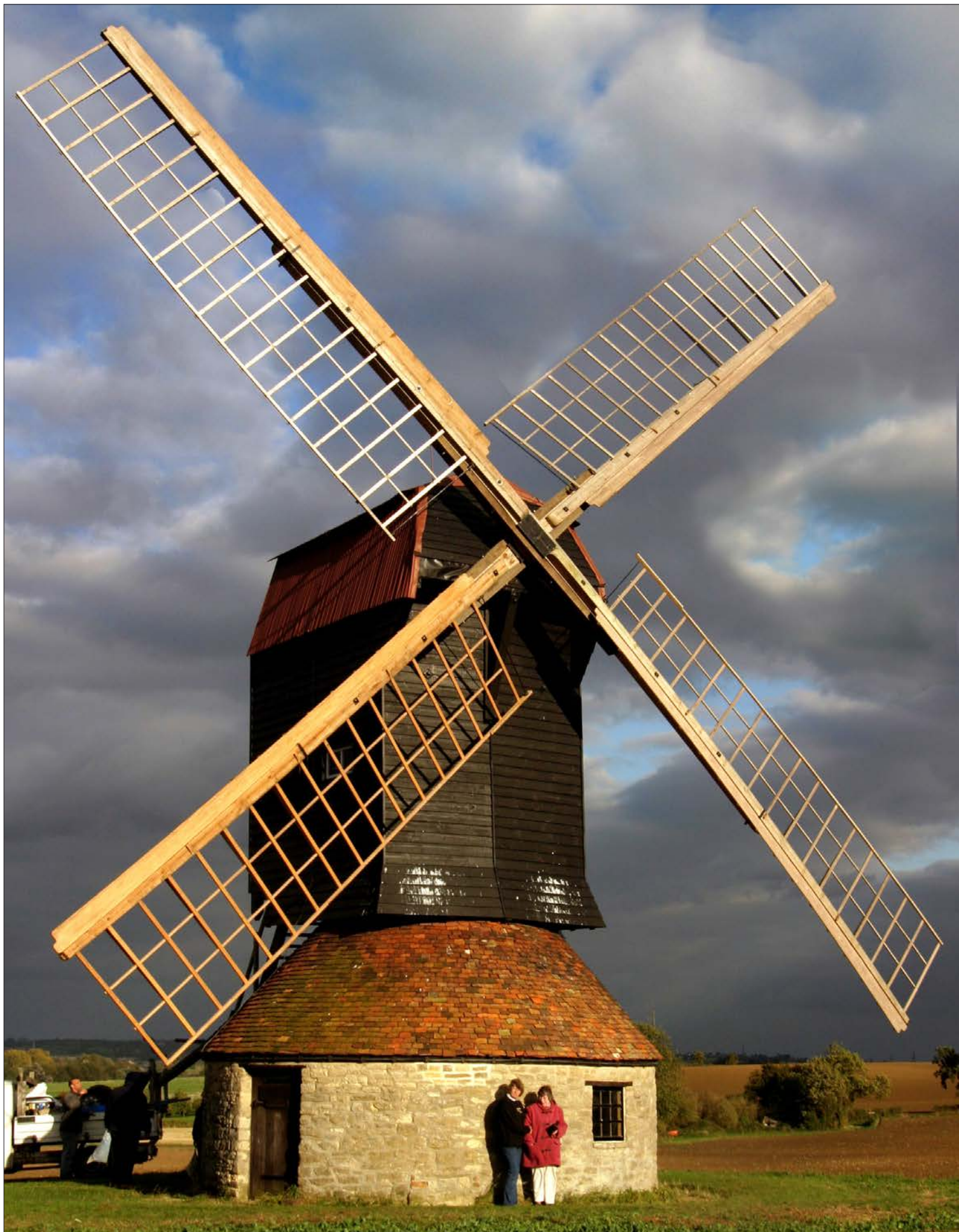
157 Mill with Sails Restored 24 September 2004
